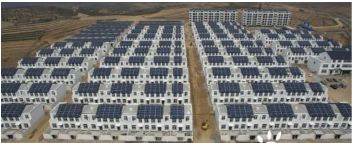
Figure 16: Jinko PV + sand control project in Northwestern China 237
